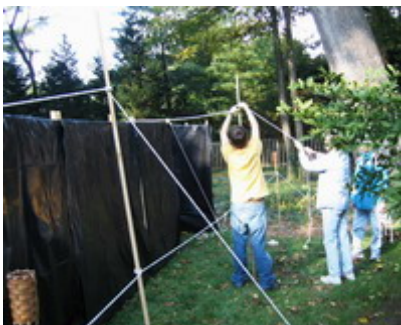
This particular design had a rope pathway outside the perimeter of the maze. So stabilization ropes (which hold panels securely in place) had to be run over the top of the pathway.
