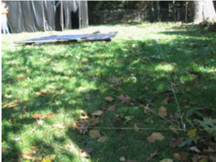
When starting the assembly, stake a twine square onto the ground to help determine where to put the panels. Use measured diagonals to make sure the square outline is truly square.
