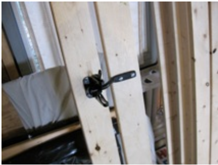
Latch detail. Be careful to line up the striker bar with the latch before bolting the bar to the door.
