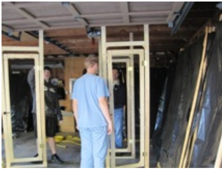
Maze doors in progress. How exciting!
