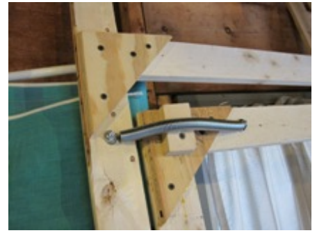
Spring detail. Note the wooden block to increase tension. Also note the spring is attached with bolts (with washers on both sides)
